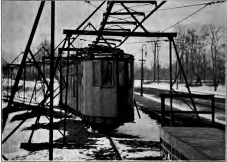
THE MONOROAD IN PRACTICAL USE FOR CARRYING PASSENGERS AT CITY ISLAND, NEW YORK
